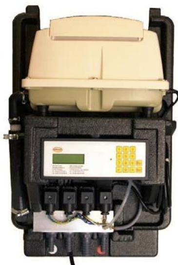
Open internal switch cabinet with hose clips
