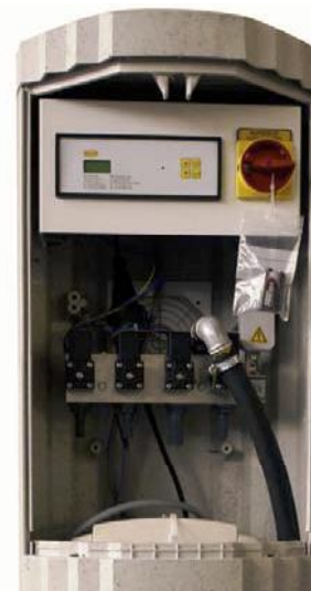
Open external switch cabinet
