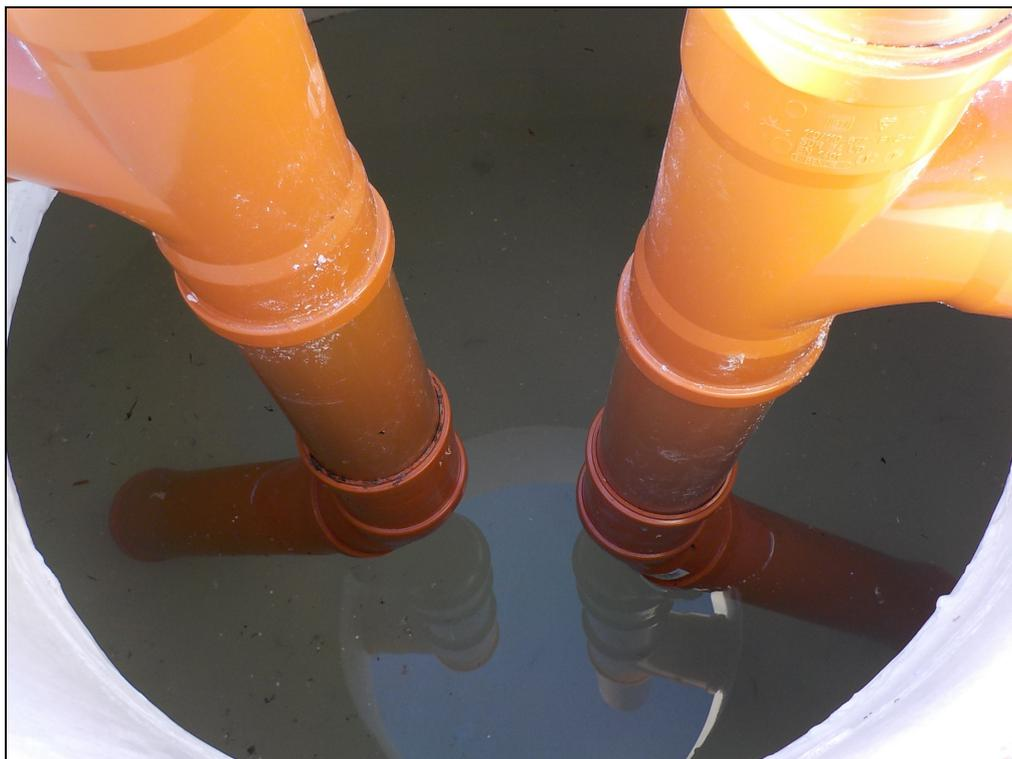
Figure 1: Inlet and outlet device
