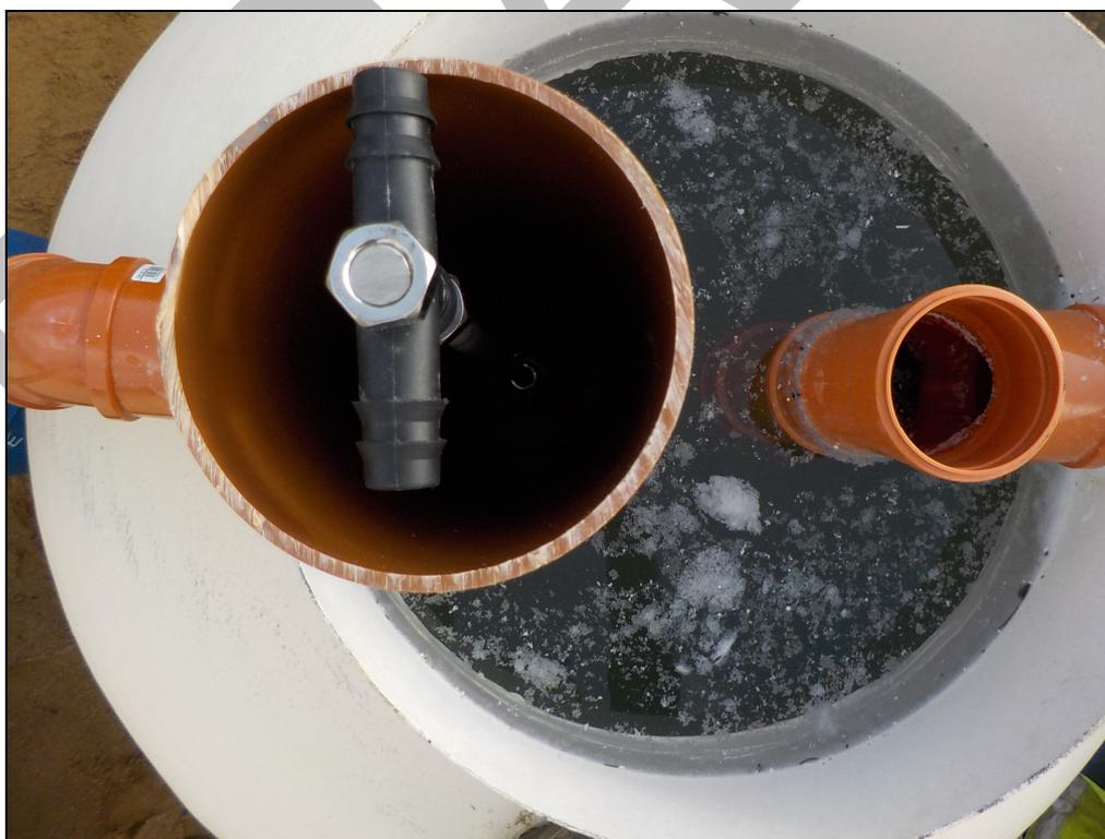
Figure 2: Outlet with filter (on the left hand side)
